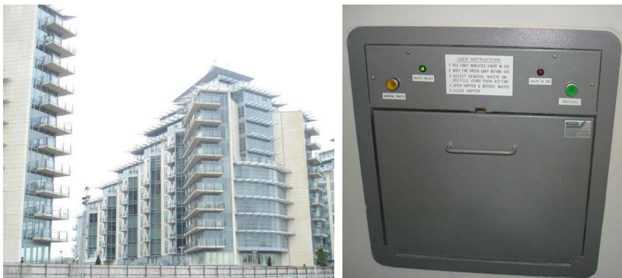
Figure E.1: Battersea Reach development and the chute inlet used
