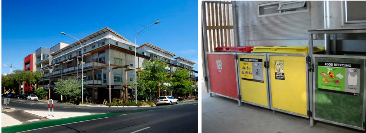
Figure E.2: Whitmore Square Affordable Eco-apartments and bins used
